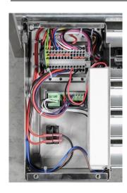
The chassis houses the connecting blocks for the refrigeration equipment, a fuse for the low power items, and a 24V dc power supply for the anticondensation heating element.
